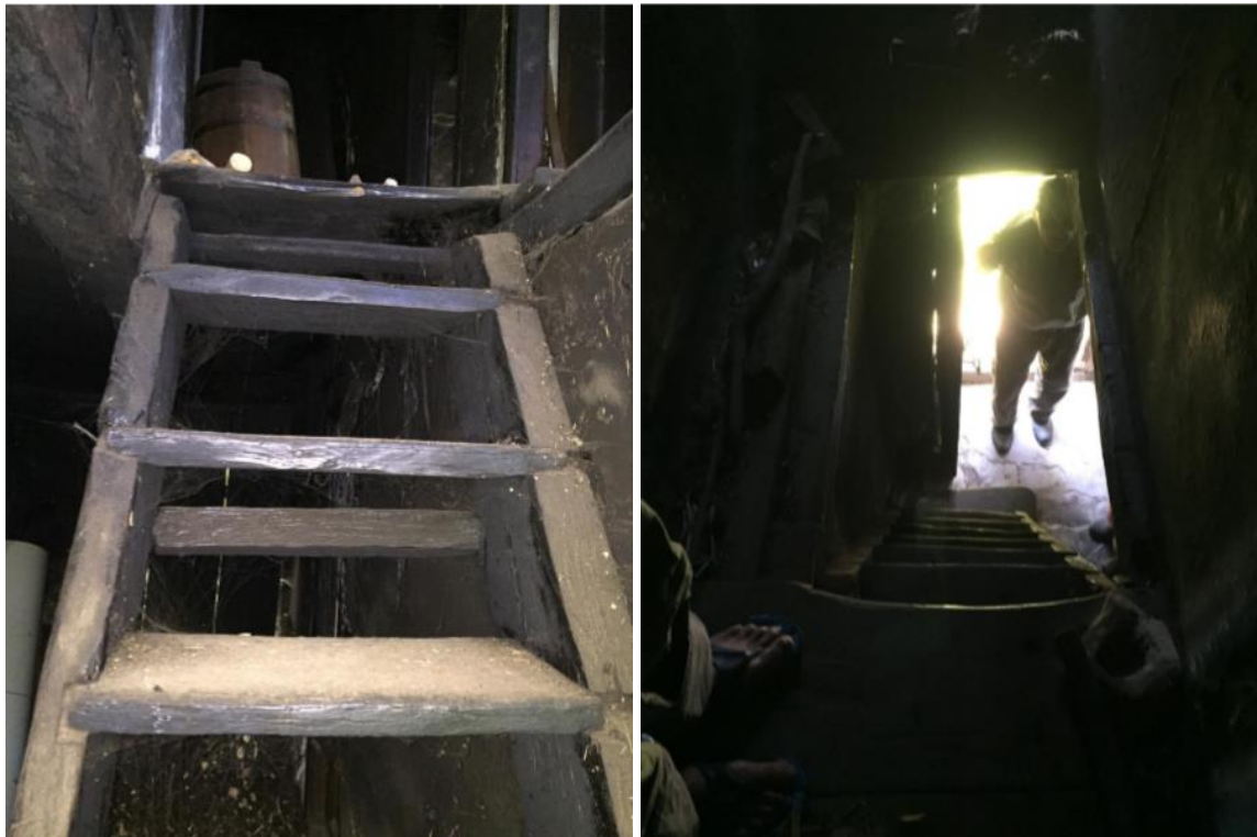
Figure 6. Staircase (basamaci) ground floor
