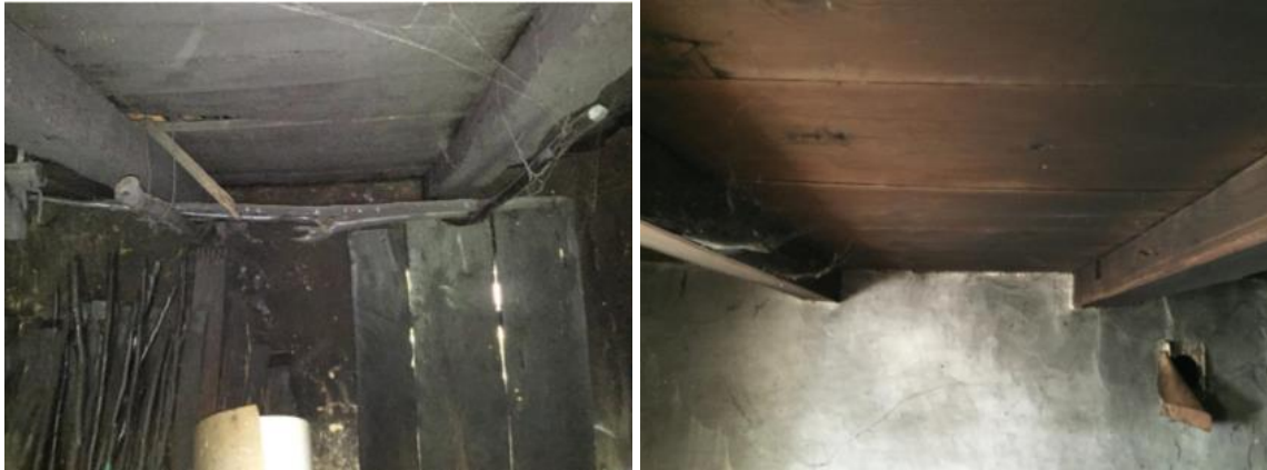
Figure 7. Ceiling construction (ground floor-first floor).
