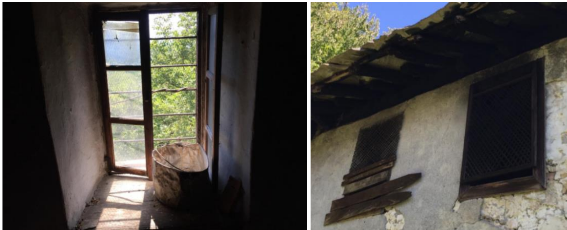
Figure 10. Window (on the main room on the ground floor).
