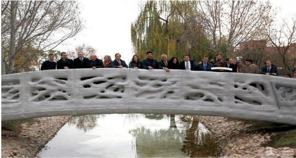
Fig. 3. 3D Printed bridge: In Spain, the first pedestrian bridge printed in 3D in the world (3DBRIDGE) was inaugurated 14th of December of 2016 in the urban park of Castilla-La Mancha in Alcobendas, Madrid.
